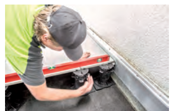
Readjustment is carried out using the large adjusting screw on the adjustable foot.
