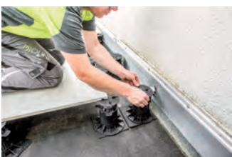
Laying the impact sound pad
