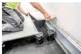
Laying the slab
