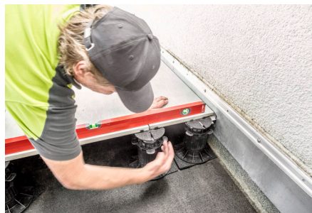
Readjustment is carried out using the large adjusting screw on the adjustable foot.
