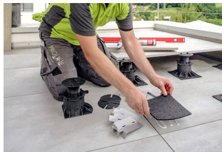
To prevent shifting under loads, the outer and corner solutions are also glued together using PU adhesive.
