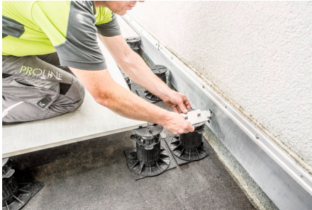
Placement of the PROSTILT clip spacer with a neoprene pad is required to prevent the slab shifting towards the wall.
