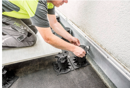
Laying the impact sound pad.
