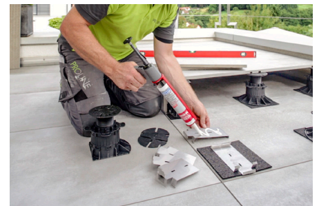
The PROSTILT clip is glued under-neath to the rubber granulate pad using the PU adhesive. In a corner location a second clip is fixed at the top overlapping at a 90° angle.
