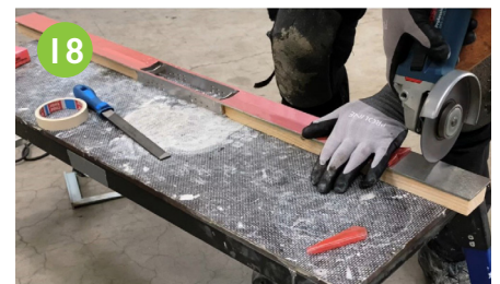
18 Separate the shower profile at the respective markings with the angle grinder and the stainless steel cutting disc (item no. 94230/94240). Caution: Only stainless steel must have been cut with the discs!
