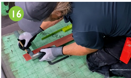
16 Use a bracket to transfer the division lines to the shower profile.
