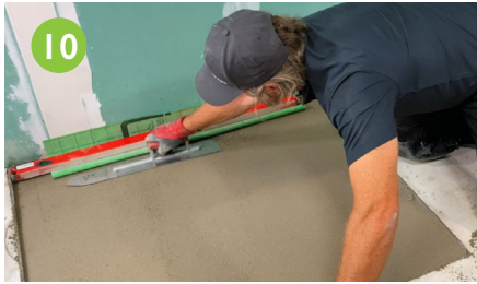
10 Plane the screed surface with the smoothing trowel.
