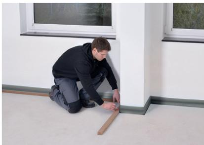
Lay the edge-insulating strips around the perimeter of the wall. Adjust the first frame support and glue it to the load-bearing substrate.
