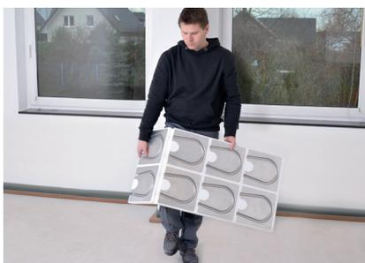
Adjust the elements using specified break-age points and fill the edge and corner areas with edge elements. Never cut the aluminium sheets!
