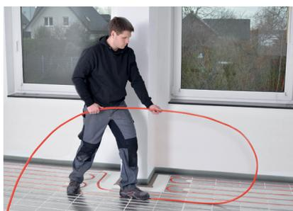
Press the multi-layer composite pipe into the pipe channels in a large arc from above without any tension. Maximum heating circuit length is 120 m.
