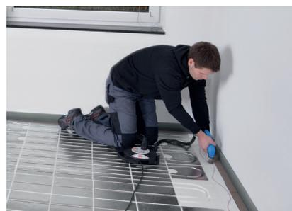
Individually cut the pipe feeds using the hot cutter: Run long pipe feeds in S-shaped paths.
