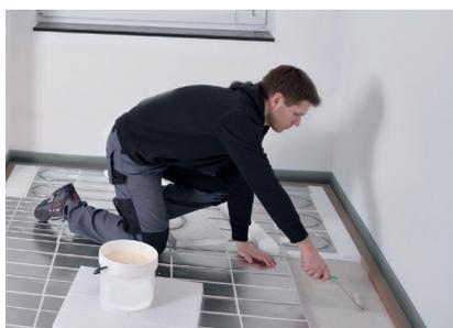
Connections on wall surfaces and compensations surfaces are filled using BasicLine edge plate and bonded across the entire surface.
