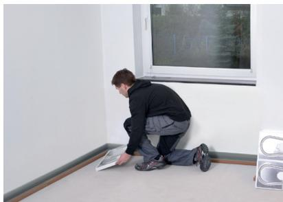
Start with the elements described according to the layout drawing and bond to the substrate over the entire area.
