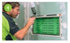
Fix and attach optionally with tile adhesive or bonding foam.
