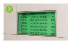
Measure the PROBOX soffits, shelf, cover and back wall and lay the tiles. Then grout and complete the silicone work in the corners.
