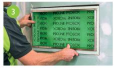
Wedge in the PROBOX with suitable material, measure and align.
