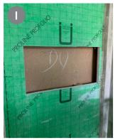
Glue the PROFOLIO sealing and decoupling film to the wall surface. Create the wall niche once tiling has been arranged and the dimensions of the PROBOX in unfinished state have been considered.
