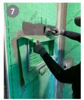
Apply PROFIX DS barrier coating around the PROBOX onto the existing seal according to width of the sealing sleeve.
