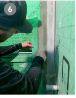
Remove excess tile adhesive. Observe the curing time of the tile adhesive.
