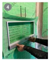
Glue in and align the PROBOX. Observe the curing time of the tile adhesive.
