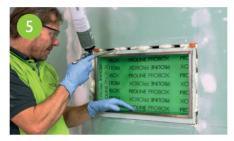
Once the fixed points have hardened, backfill and trowel off the assembly space.
