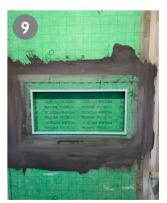
After the PROFIX DS has hardened, the PROBOX is ready for tiling.
