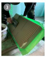
Spread tile adhesive on the back of the PROBOX.
