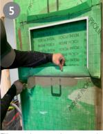
Fill up the gap between the PROBOX and the sealing level below the sealing sleeve all around with tile adhesive.
