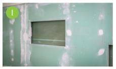
Create the wall niche once tiling has been arranged and the dimensions of the PROBOX in unfinished state have been considered.
