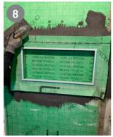
Insert the sleeve into the PROFIX DS without creating any creases. Use a suitable scraper or trowel to press in the PROBOX sealing sleeve without creating any creases and smooth any emerging excessive PROFIX DS over and along the edge of the adhesive joint.
