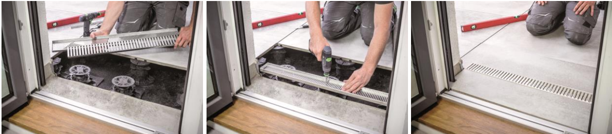
Caption: Installation of the PROSTILT drainage channel set in accordance with DIN18040-2
