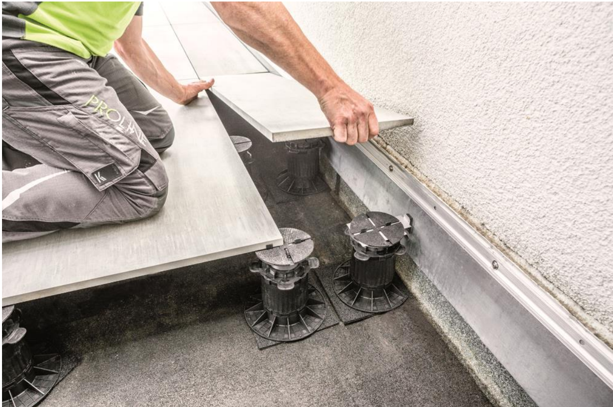
Caption: Safe and reliable laying of outdoor ceramic tiles and natural stone on roof terraces using PROSTILT
