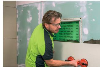
Measure the PROBOX soffits, shelf and cover as well as back wall and lay the tiles.
