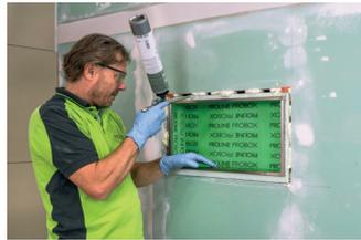
Once the fixed points have hardened, backfill and trowel off the assembly space.
