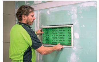
Wedge in the PROBOX with suitable material, measure and align.
