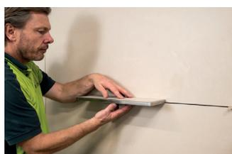
Cut the tiling to size and stick it on. Grout and insert the silicone joint once dried.
