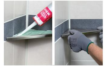
Apply OTTOCOLL M 500 or tile adhesive to the area of the PROSHELF to be tiled. Then place the tiles that have already been cut to size.
