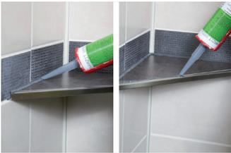
Seal the newly created joints with permanently elastic and neutrally interconnecting silicone.
