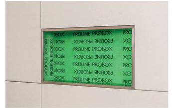
Then grout and complete the silicone work in the corners.
