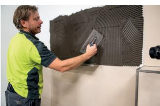
Continue with laying the wall tiles. Rework the whole side surface at the top with tile adhesive.
