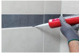
Apply OTTOCOLL M500 hybrid adhesive and sealant to the cleaned joint gap.
