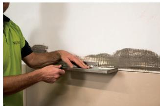
Remove excess tile adhesive in the installation area. Push the PROSHELF with the bottom side surfaces behind the tiling.
