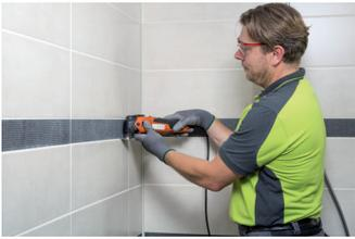
Remove the joint with a suitable tool (e.g. angle grinder) and clean.
