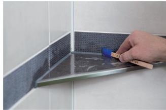
Strip and smooth the silicone joints using a suitable joint smoother.
