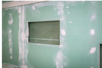
Create the wall niche once tiling has been arranged and the dimensions of the PROBOX in unfinished state have been considered.
