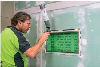
Fix and attach optionally with tile adhesive or bonding foam.
