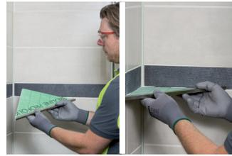
Place the PROSHELF in the joint gap that has been filled with adhesive (slight gradient forward recommended).
